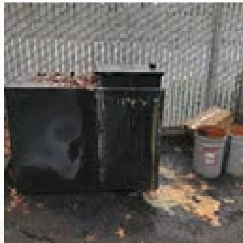
Before: Same photo from a different angle. You can see the clear signs of spillage on the container itself and the ground next to the container.
