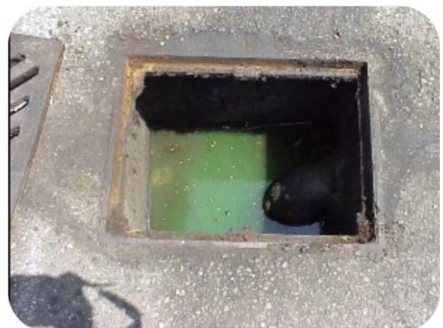
Radiator fluid (photo courtesy Federal Way)
